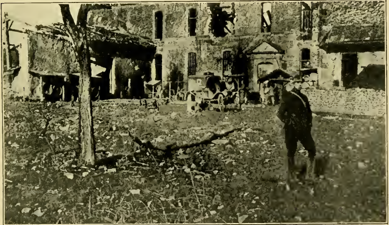
THE COURTYARD OF THE ESNES CHÂTEAU
